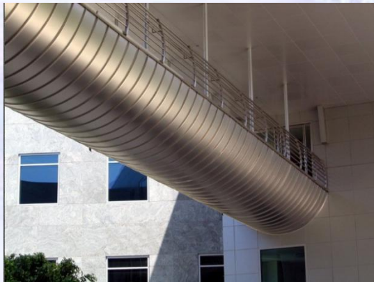
Medical Building Pedestrian Bridge Beverly Hills, California
