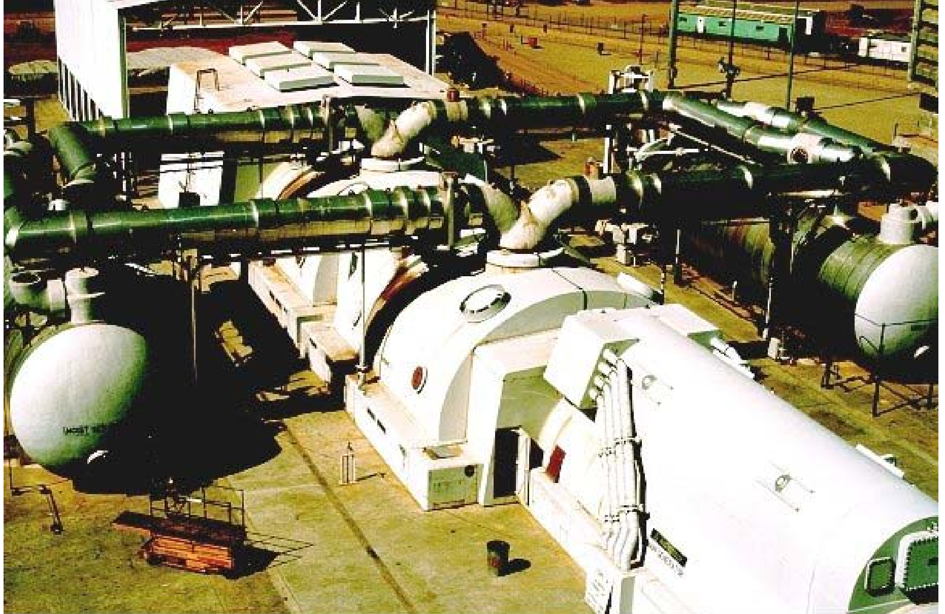
Overview of a steam turbine and main generator for a nuclear steam power station. (Courtesy of Carolina Power and Light Company)
