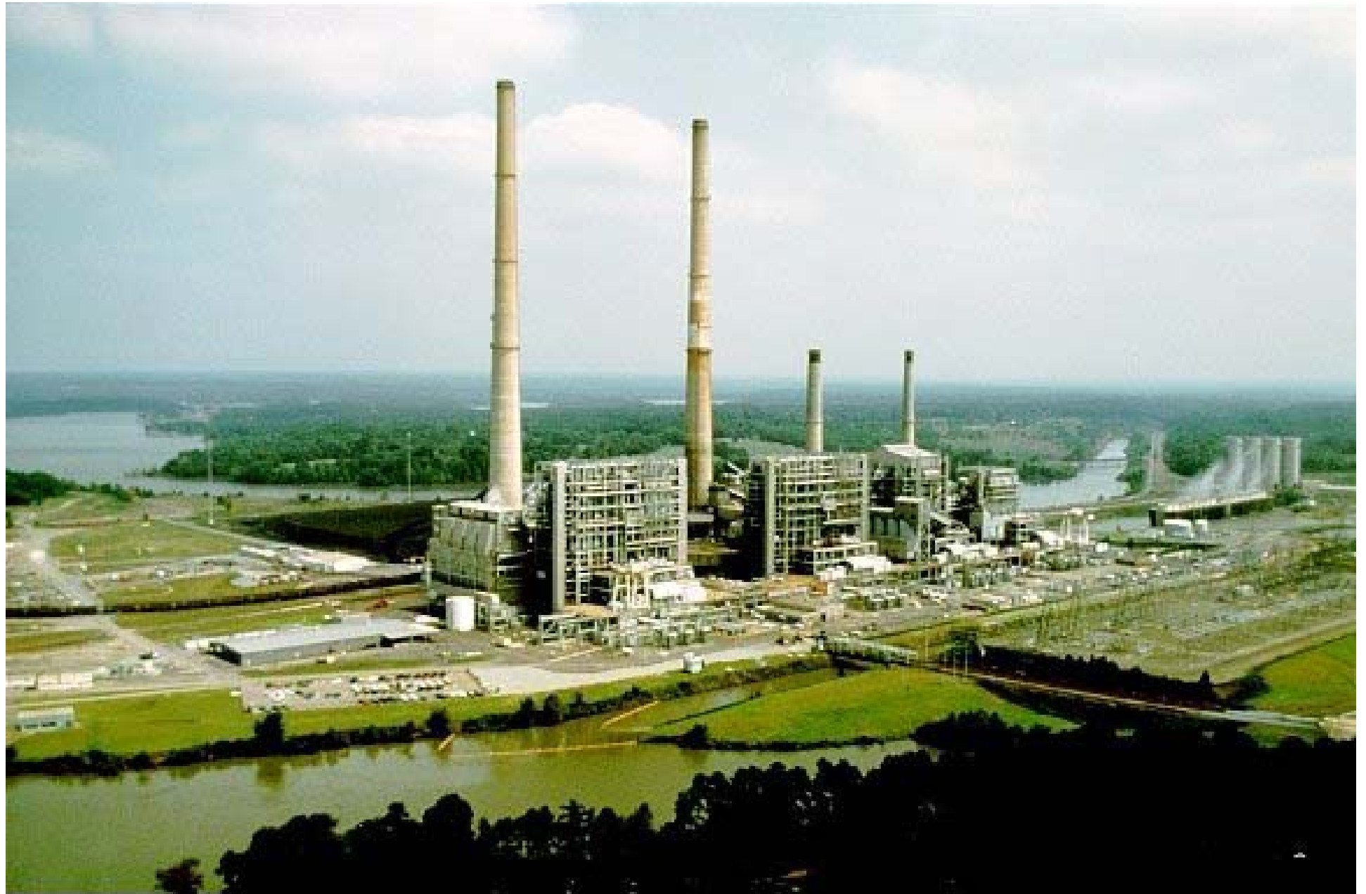
Overview of a coal fired steam power station. (Courtesy of Carolina Power and Light Company)
