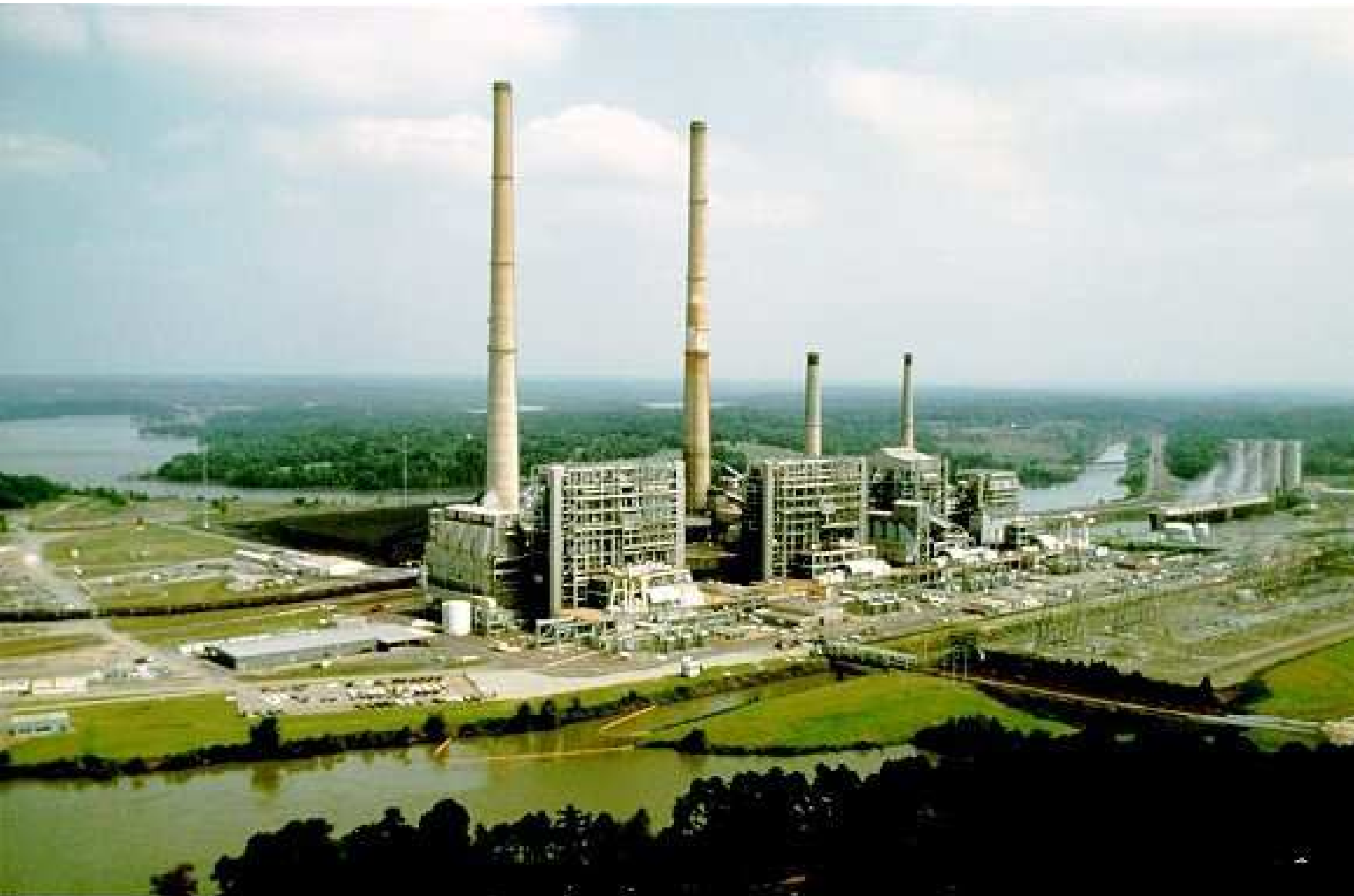
Overview of a coal fired steam power station. (Courtesy of Carolina Power and Light Company)
