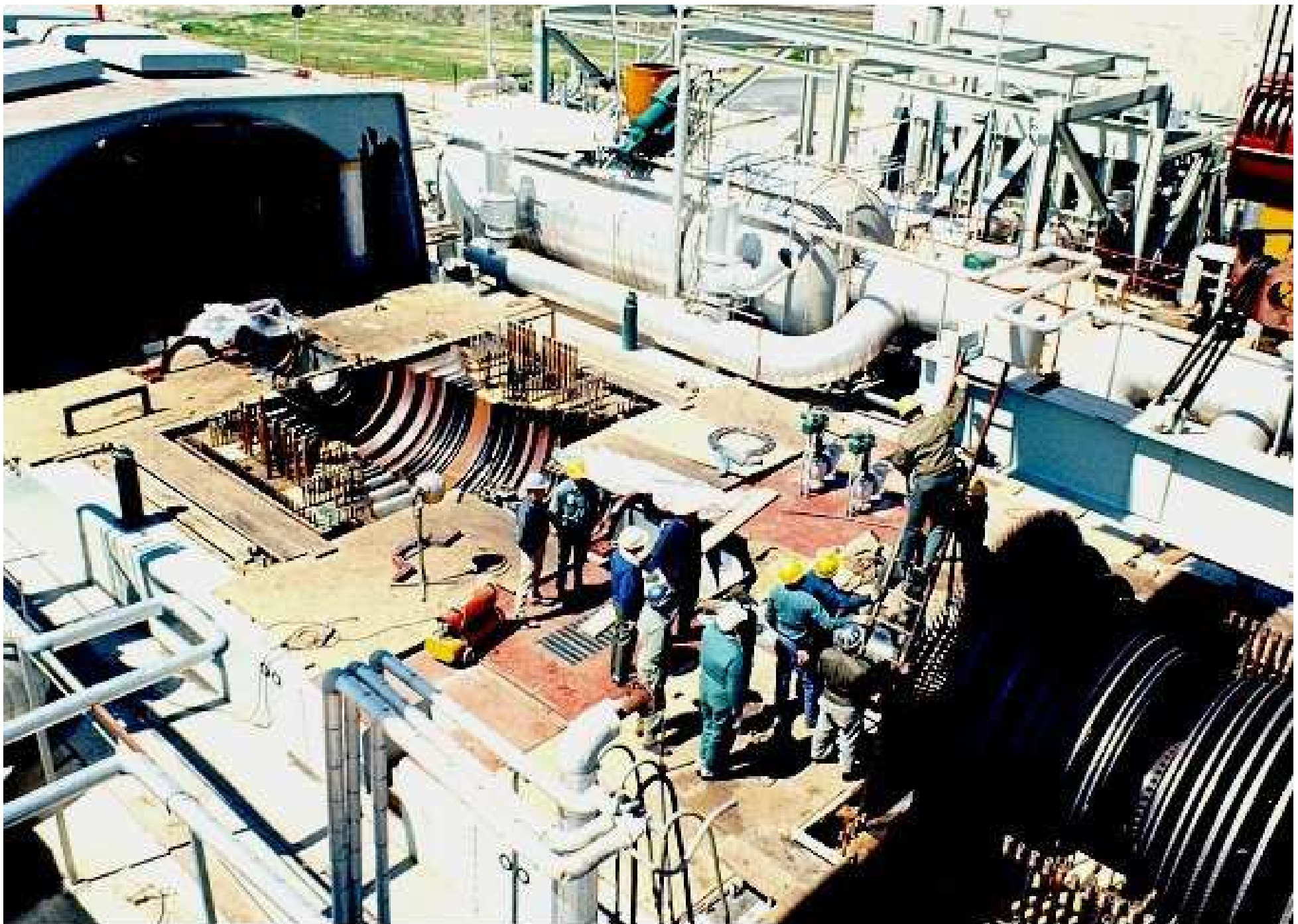
Turbine bed for a steam power station. (Courtesy of Carolina Power and Light Company)
